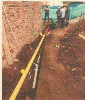
TUBERIA PVC/SANT Ø 2" TUBERIA PVC/ALL Ø 3"
