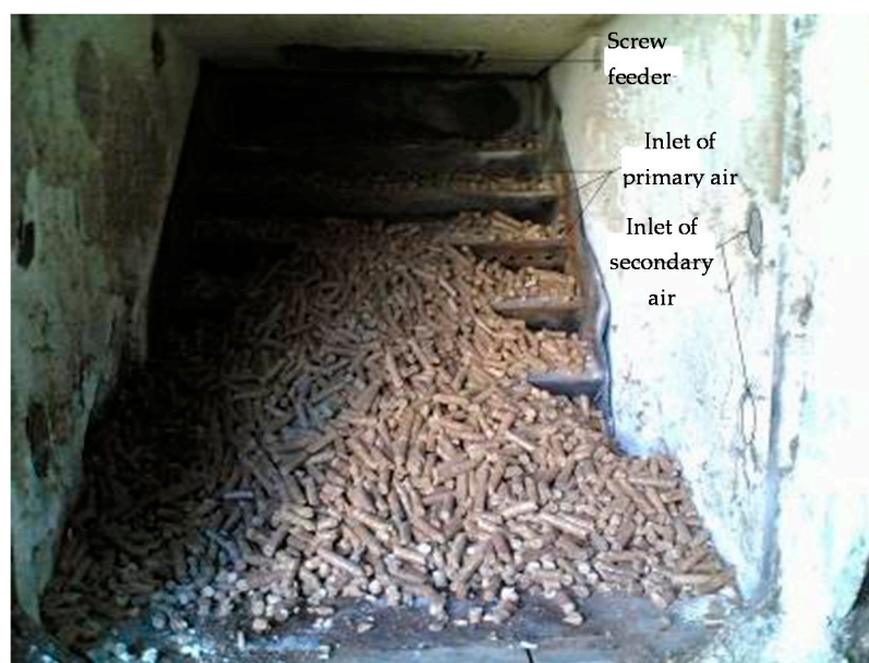
Figure 9. Filling of BIO System burner with pellets from almond tree.
