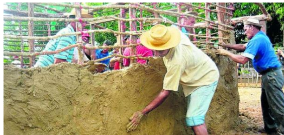
Figure 3. Bahareque wall construction, Villa de los Santos Source: Alcibiades Cortez
