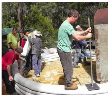
Figure 5. Rammed earth bags Source: Comencemos una Ecoaldea
