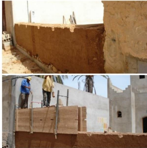
Figure 2. Construction rammed earth wall– Marruecos
